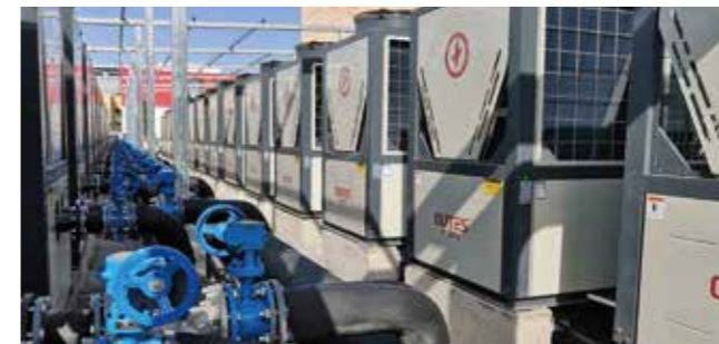
Liaoning Province Dalian City Vocational Technical School Heating Area: 150, 000m 2 Heat Pump: mixed models Total: 78Units
