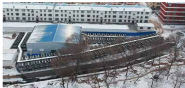
Helingeer Town, the Nei Monggol Autonomous Region Heating Area: 100, 000m 2 Heat Pump: 150kW/unit Total: 80Units
